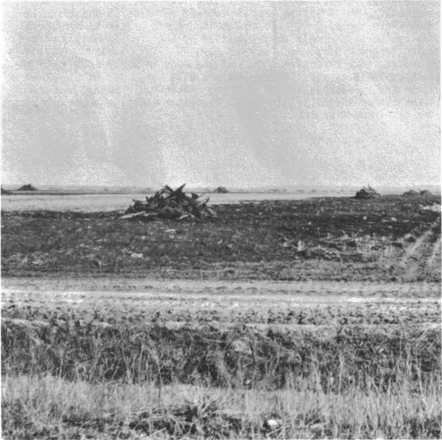
Figure 15. Windrows repiled after initial burning to separate the soil from the remaining wood and facilitate reburning.
