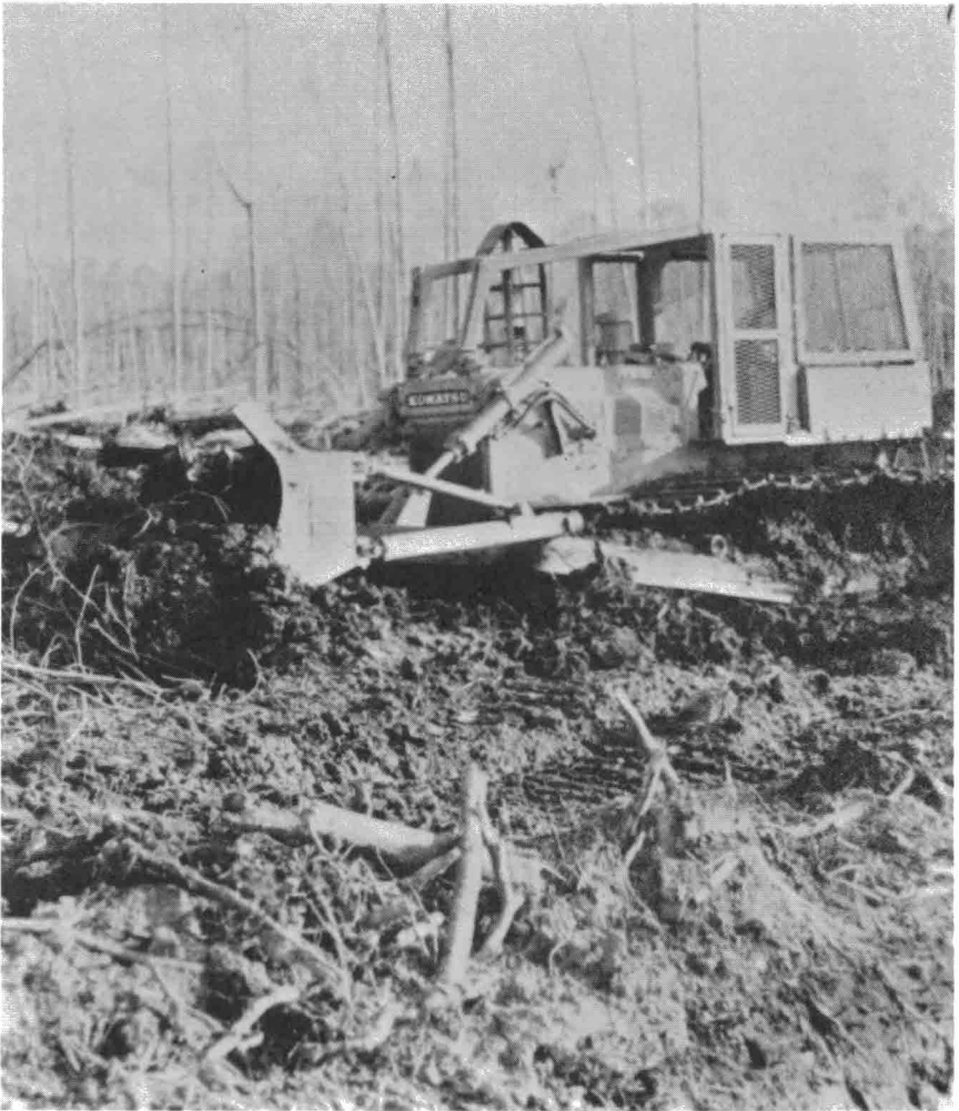
Figure 13. Spoil from the field ditch being moved toward the center of the field during the land clearing process.
