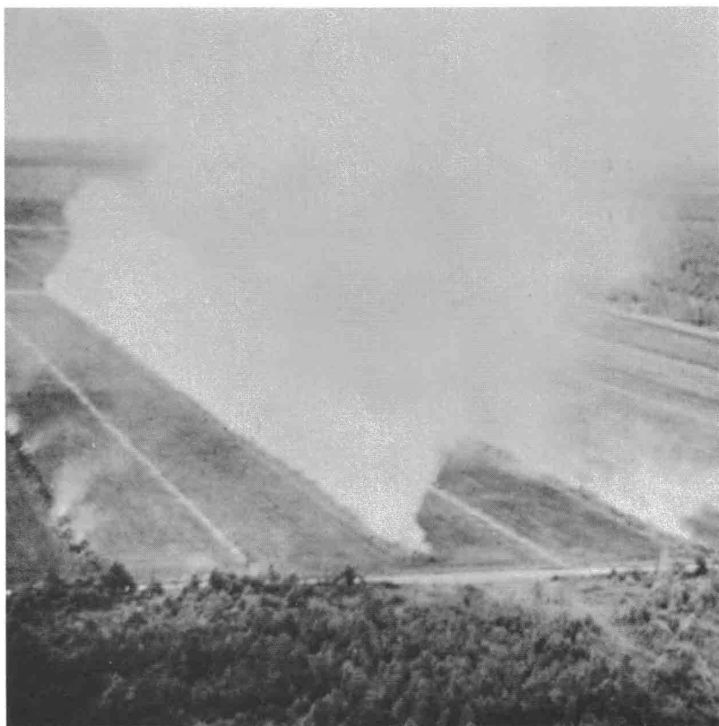
Figure 14. Windrows being burned to eliminate woody debris.
