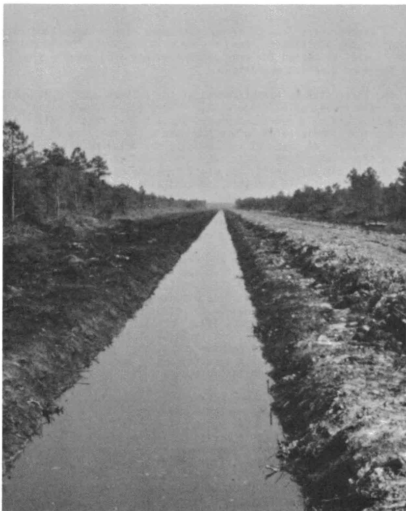
Figure 10. Primary canal system being dug as the first step in land clearing and development.
