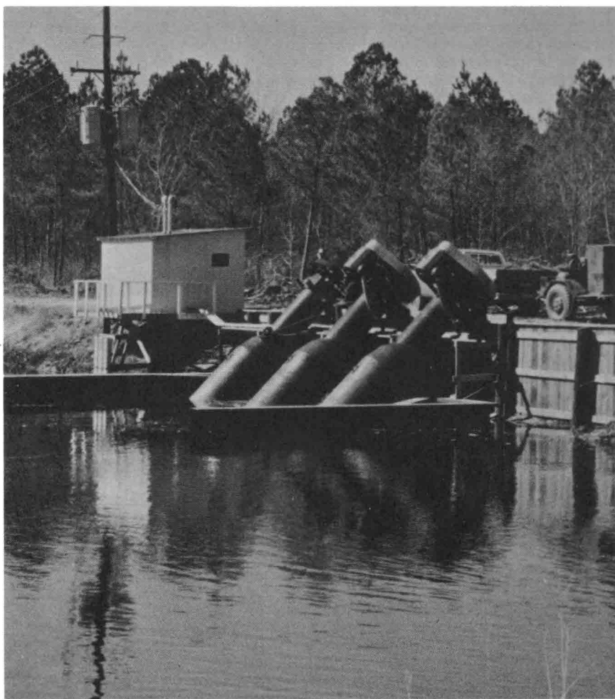
Figure 20. Pumping station with tide gates to remove excess water from low-lying farm land.
